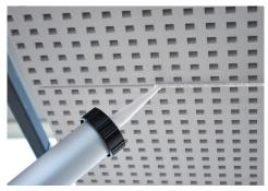
The material itself is ready for use and has creamy consistency. In order to reduce the risk of subsequent crack formation, the joint compound is fibre-reinforced and boasts very high density.
